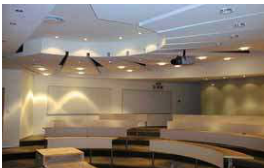
▼ Typical ceiling application showing recess features and bulkheads.
