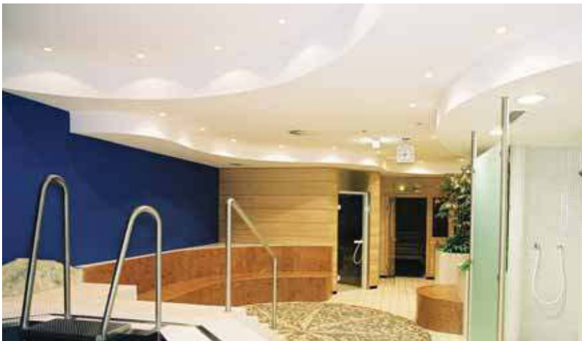
▼ Typical ceiling application showing curved bulkheads.
